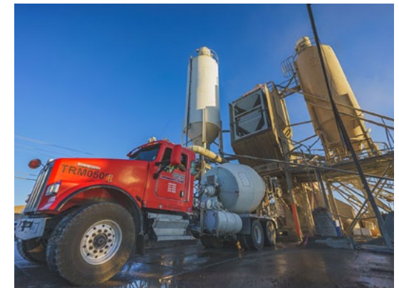
American Ready-Mix Plant, Moundhouse, NV.
